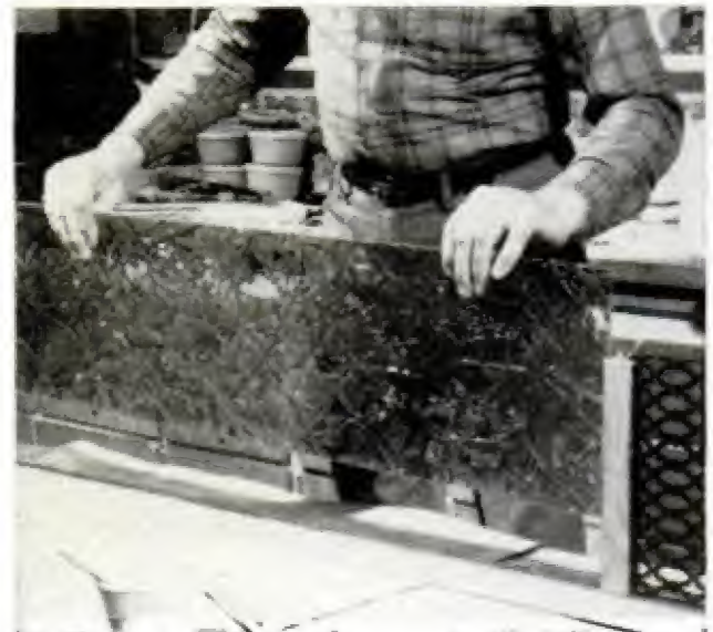
FOR NEAT JOB , paint the grooves before installing plastic. Use a few drops of glue for added strength
